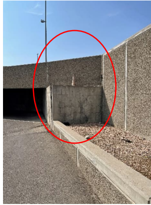
Figure 1 - Subject retaining wall (scope).
